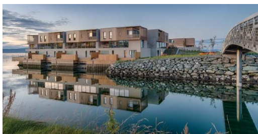
Moelven Wood Prosjekt AS supplied the facades in untreated cedar to the project "Grilstad Marina" in Trondheim. (Photo: Matthias Herzog)
