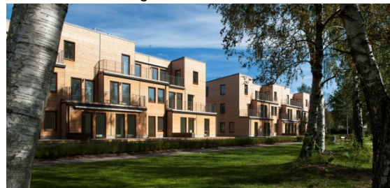
Climate smart construction and architectural innovation in the project "Ångsnäs Terrass" in Huddinge. Building modules supplied by Moelven Byggmodul AB.
