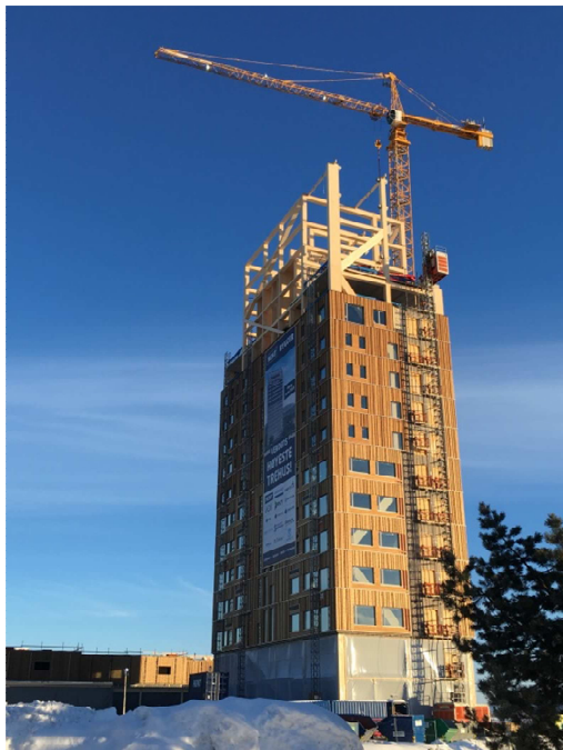
«Mjøstårnet» in Brumunddal is already before completion the world's tallest wooden building. When completed, the building will be more than 80 meters tall and an international landmark building. (Photo: Rune F. Andersen)
