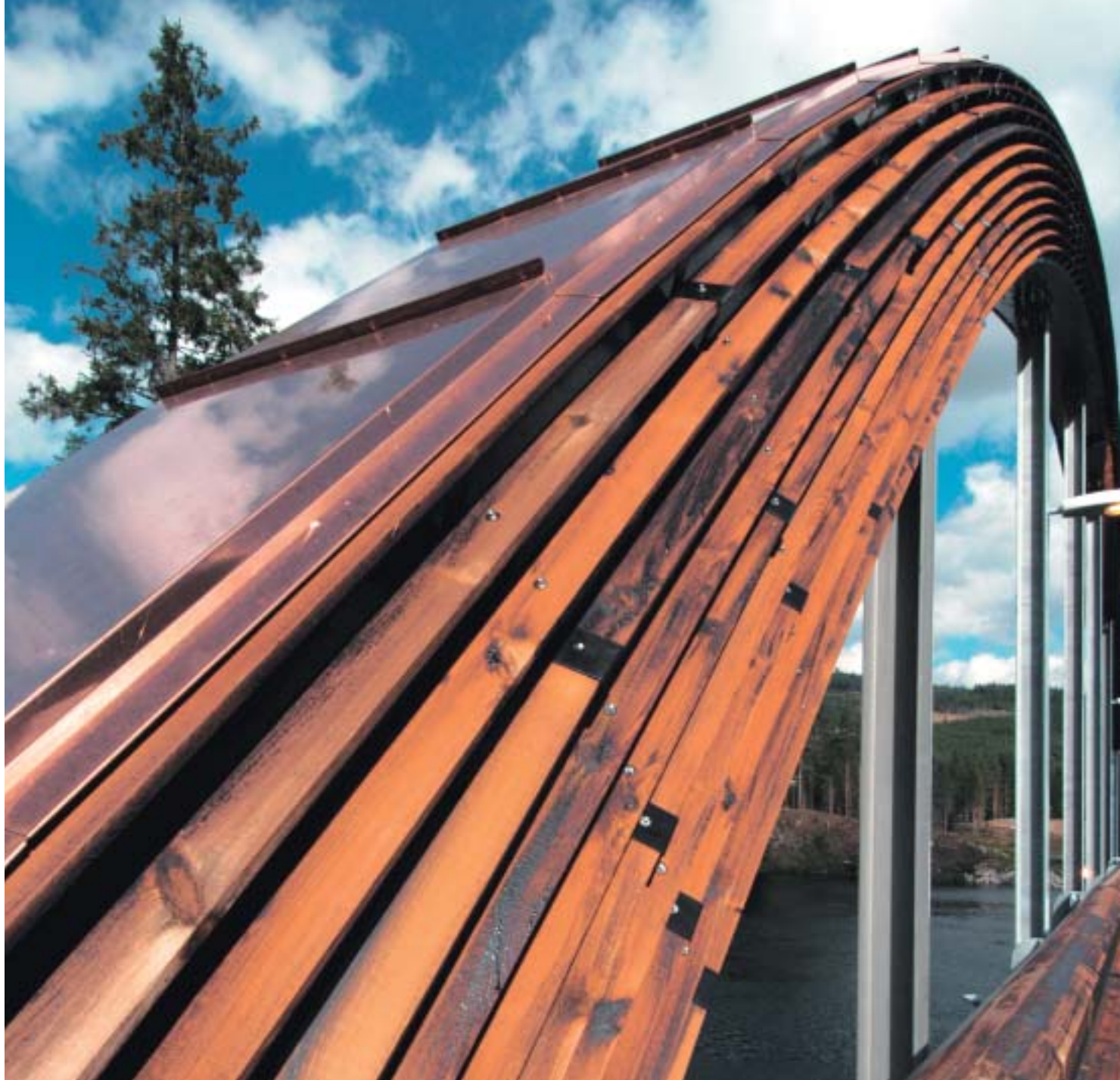
Nybergsund bridge with laminated timber structures from Moelven Limtre AS.
