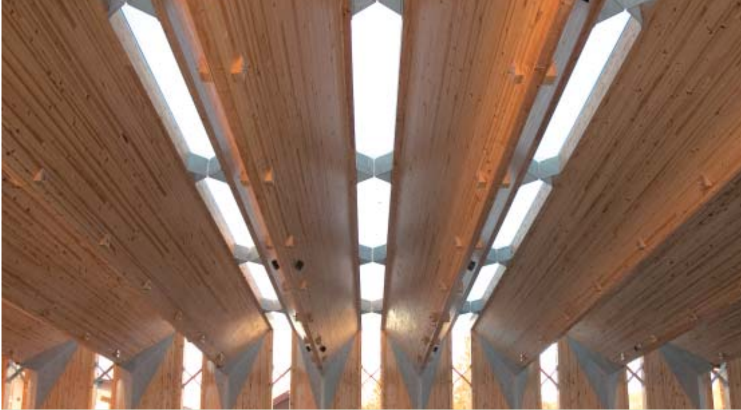
New-build at Hedmarksmuseet with laminated timber from Moelven.
