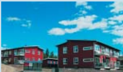
BoKlok apartments at Fagerstrand, Oslo
